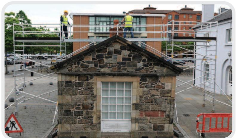
Spandeck links 2 towers for chimney maintenance in Belfast.
